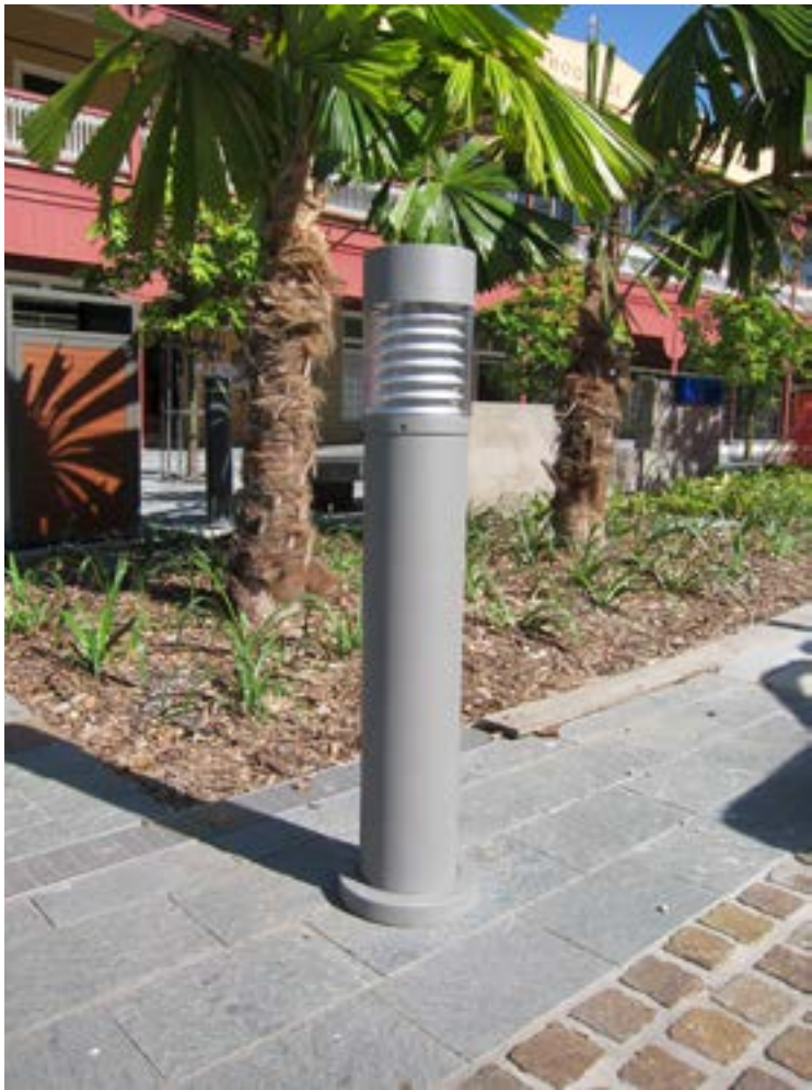
Example of an existing Light Bollard on Lake Street
