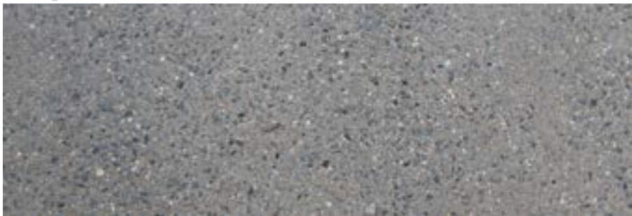
Water Washed Coloured In-situ Cast Concrete
