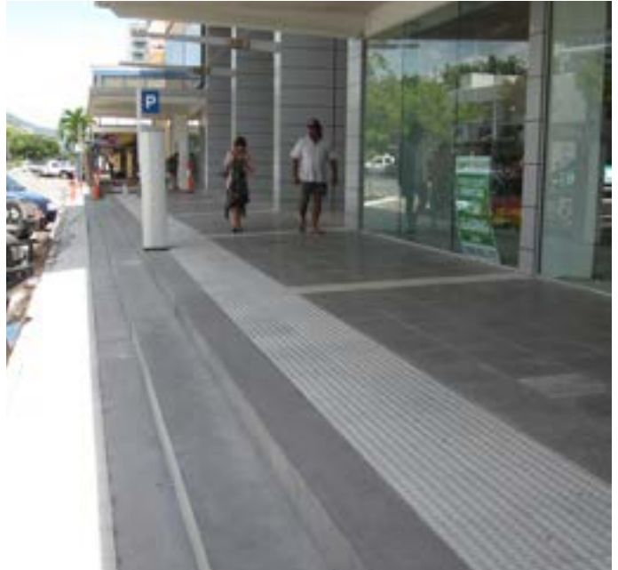
Example of kerb-side steps.
