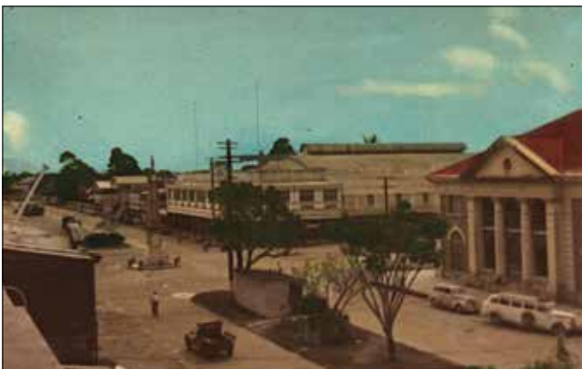
The air-raid shelter in the middle of the street
