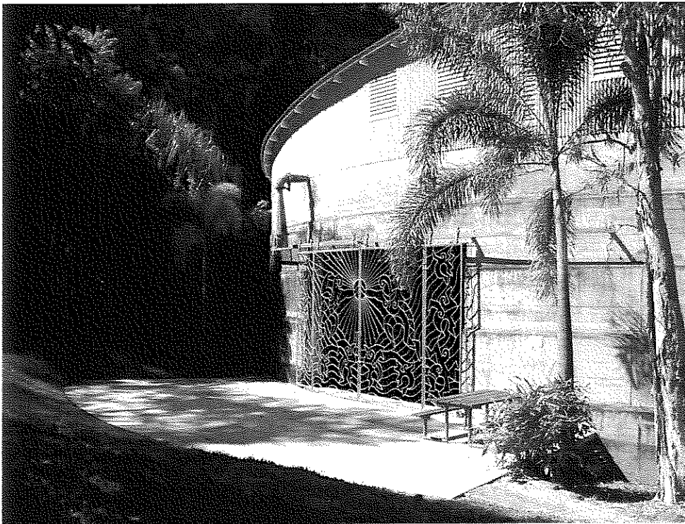
Plate 12 The small stage area outside Tank 3. The sloping earthen bund wall forms seating and a convenient amphitheatre.
