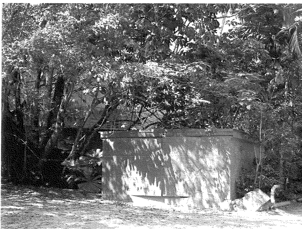
Plate 18: One of the two remaining foam sheds (this one outside tank 5).
