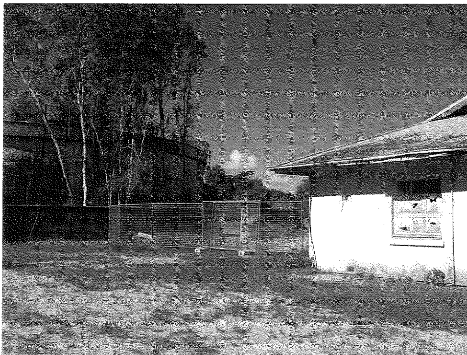
Plate 17: Tank 2 and the associated pump house.
