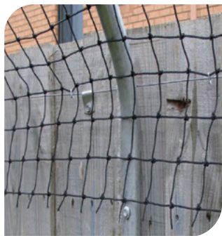
Figure 6. Netting affixed to fencing with wire
