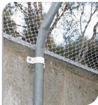
Figure 7. Netting affixed to fencing with brace
