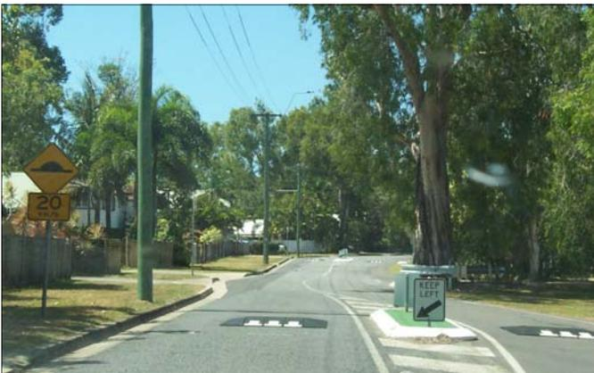
Figure 2—Rubber speed cushions with raised concrete centre kerb
