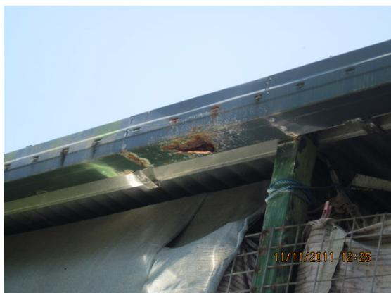
*Rusted and damaged guttering can cause a nuisance or damage to neighbouring allotments. All guttering and downpipes are to remain in good repair and condition*
