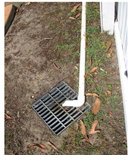
*An inter allotment drainage pit can be used in your yard to direct excess ground water to the lawful point of discharge.*
