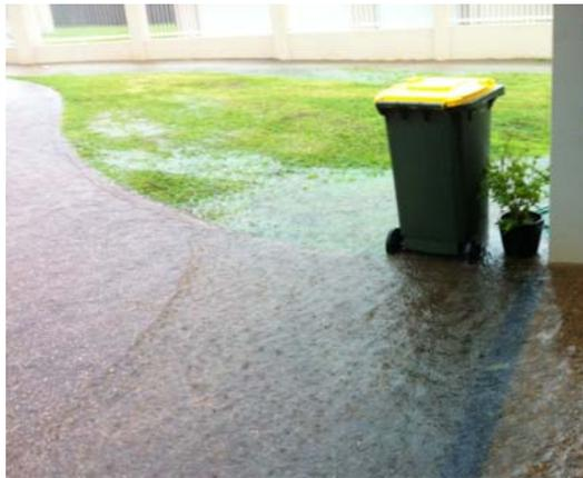
*Ground water inundation due to the contours of the land. In this case inter allotment drainage pits would need to be constructed at the top of the bank to collect the water to prevent inundation of the dwelling.*
