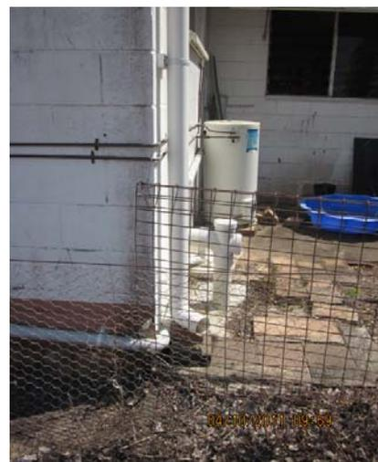
*Roof stormwater pipes not connected to approved stormwater outlets can cause damage to your property and neighbouring properties.*
