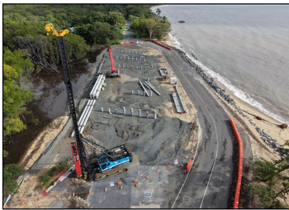
Casuarina Street Bridge (detour road)
