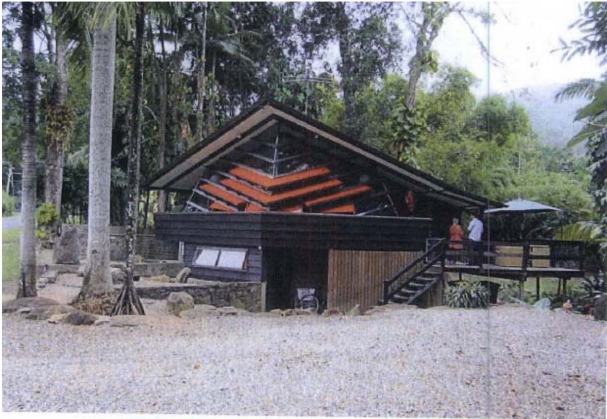
Figure 2: View of Studio from the south (Source: EHP site visit 28/06/12)
