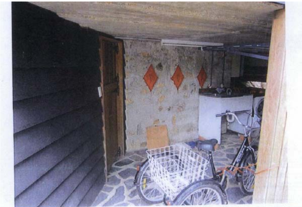
Figure 7: Lower level, showing original concrete and stone walls and later weatherboard enclosure (Source: EHP site visit 28/06/12)
