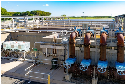
Wastewater Treatment Plant (Trunk)
