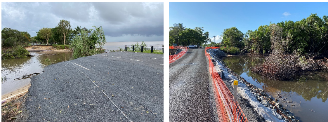
Pictured: Casuarina St Holloways with temporary causeway
