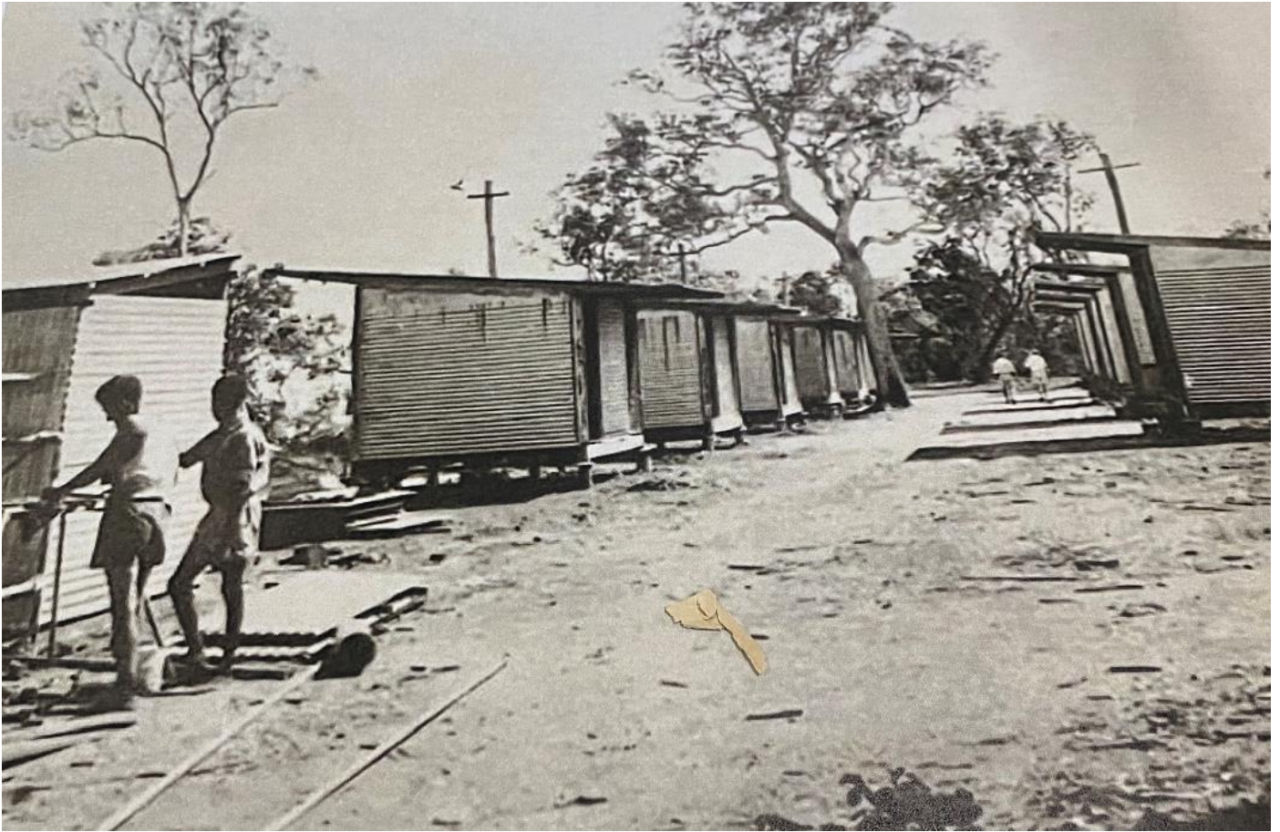
Construction of prefabricated worker accommodation in Weipa.
