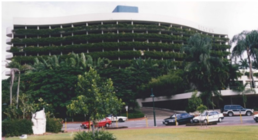
Figure 4.7.e – Example of vertical landscaping – Cairns Hilton
