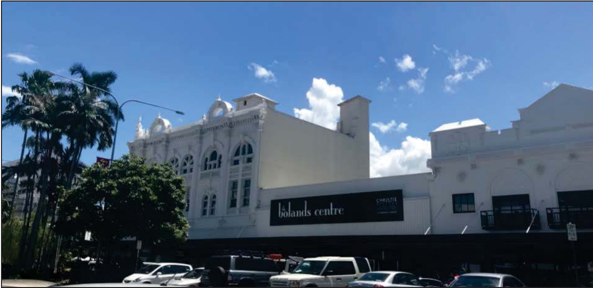
View of the streetscape and Bolands Centre from Spence Street
