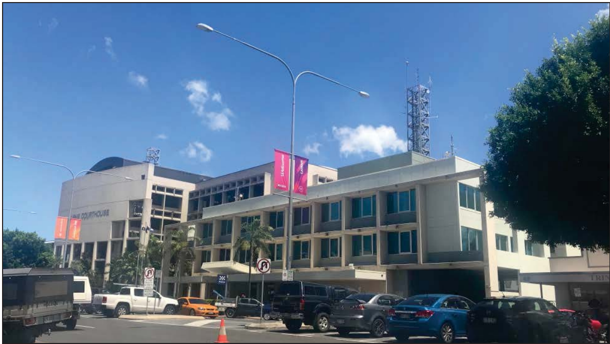
View of the streetscape from Sheridan Street
