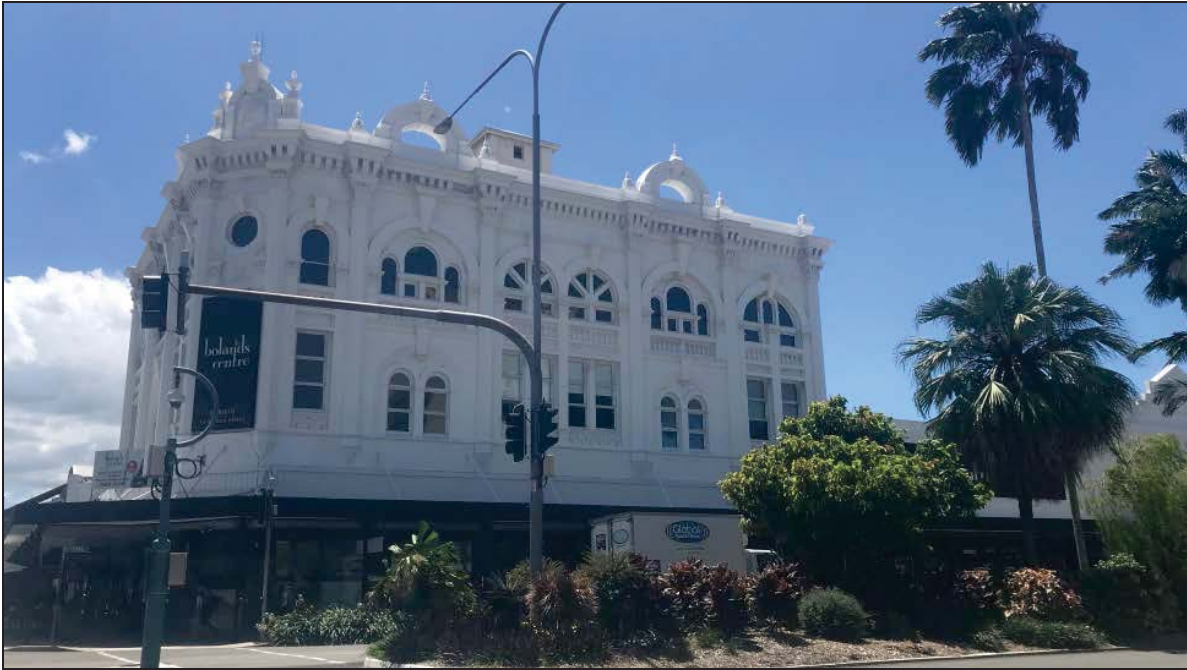
View of the streetscape and Bolands Centre from Spence Street
