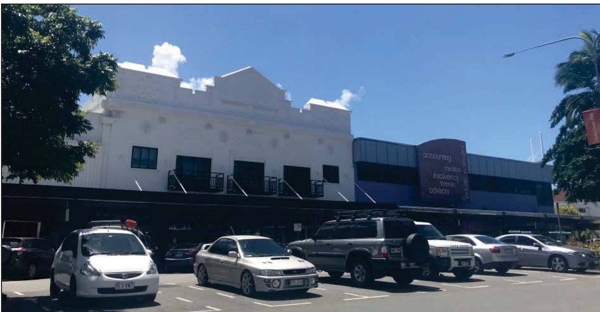
View of the streetscape and Bolands Centre from Spence Street
