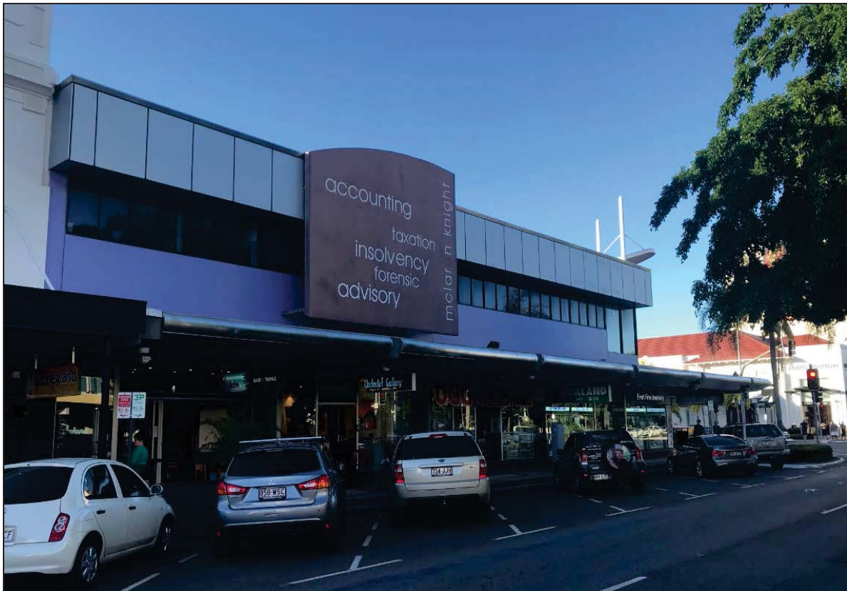
View of the site from Spence Street
