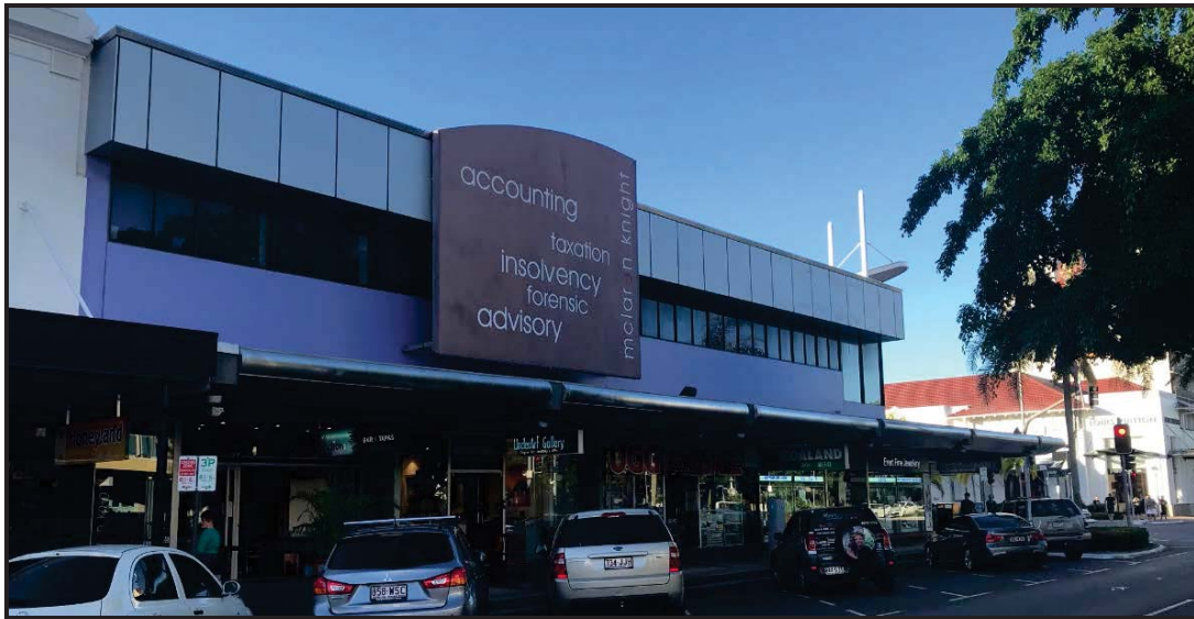
Photo 1: View of the site from Spence Street (looking eastward)
