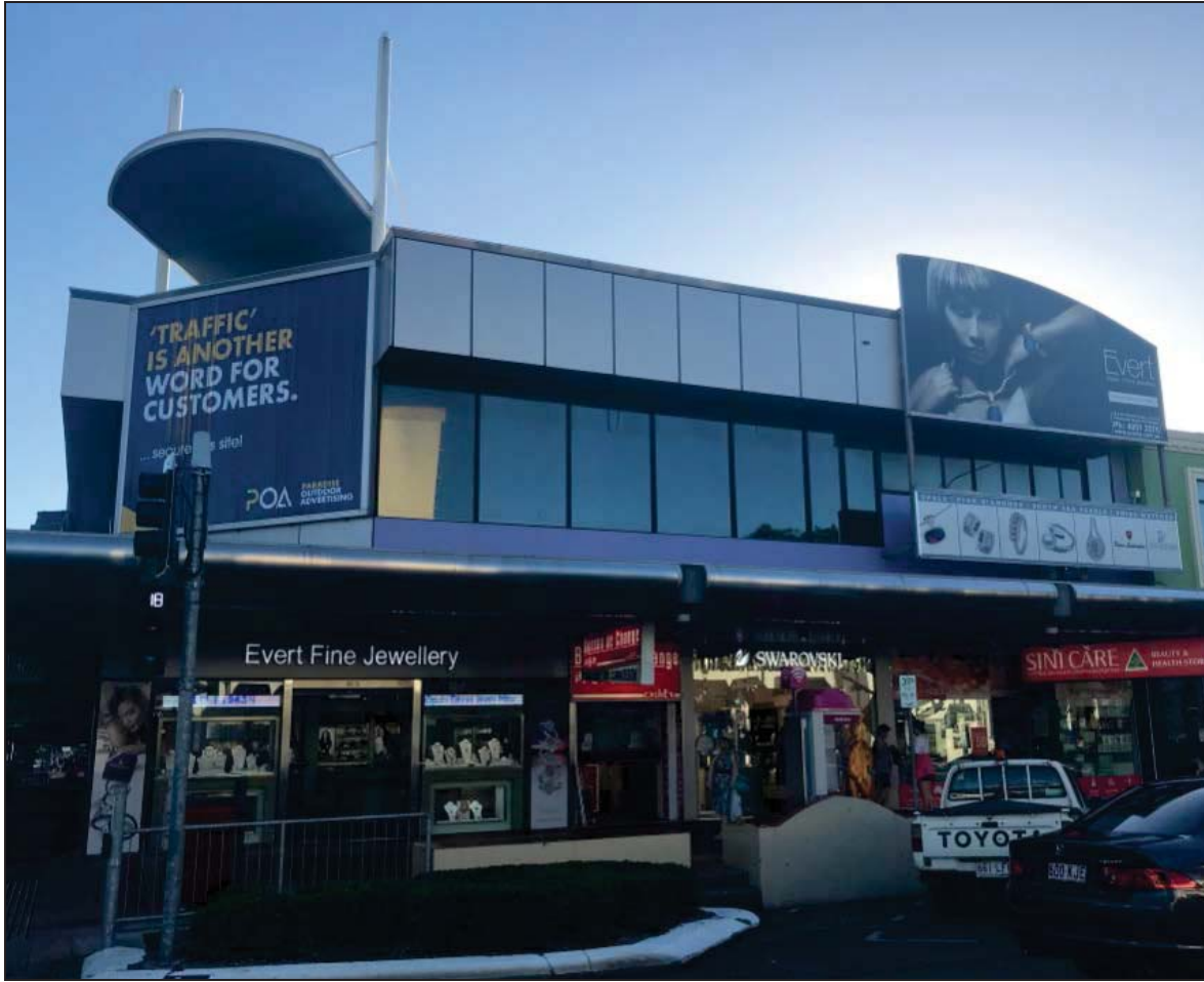
View of the site Abbott Street
