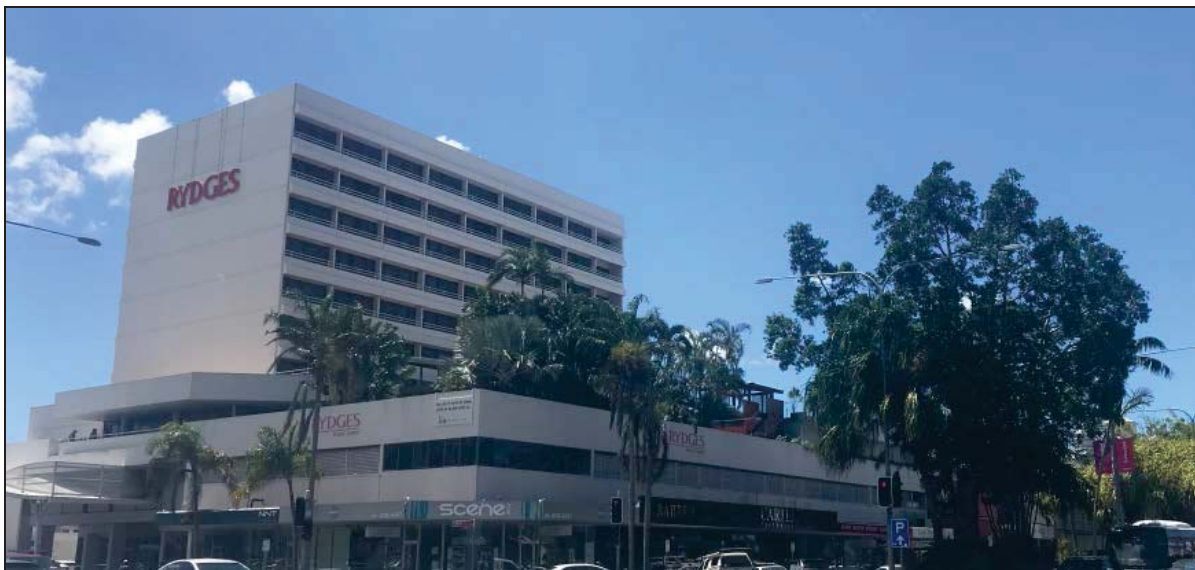
View of the streetscape from Spence Street
