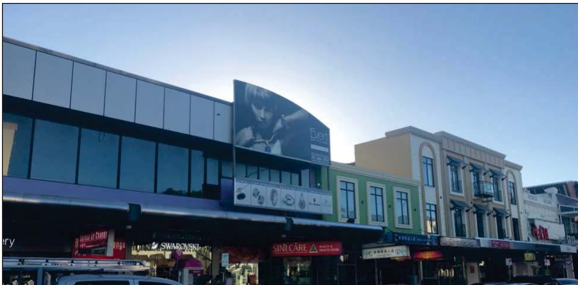
View of the site Abbott Street
