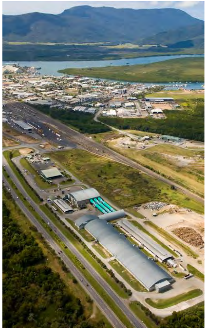
Advanced Resource Recovery Facility (Bedminster), Transfer Station and Buy Back Shop
