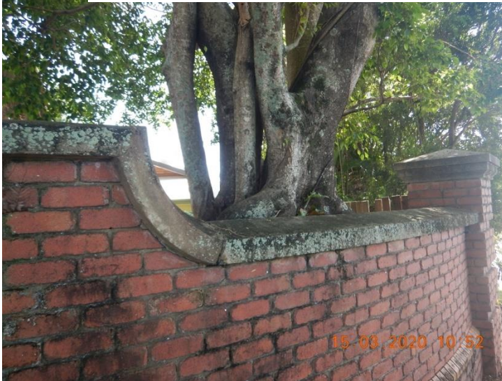
Damage being caused to City View Estate entry statement wall by Fig tree
