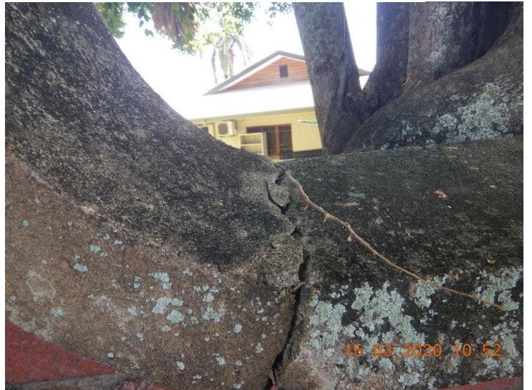
Damage being caused to City View Estate entry statement wall by Fig tree
