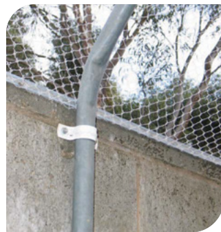
Figure 7. Netting affixed to fencing with brace
