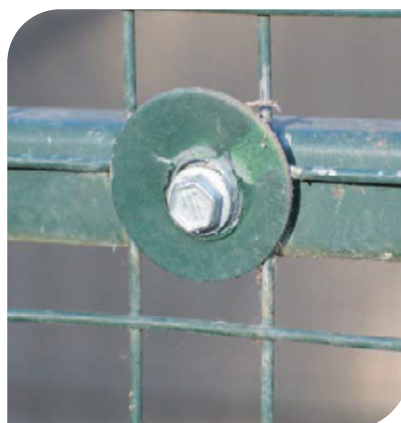
Figure 5: Fixing light mesh
