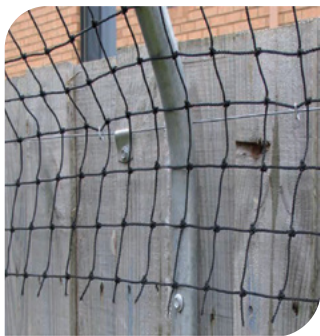
Figure 6. Netting affixed to fencing with wire
