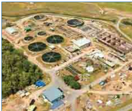
Aerial photo of the Northern Treatment Plant – top of Greenbank Road, Aeroglen
