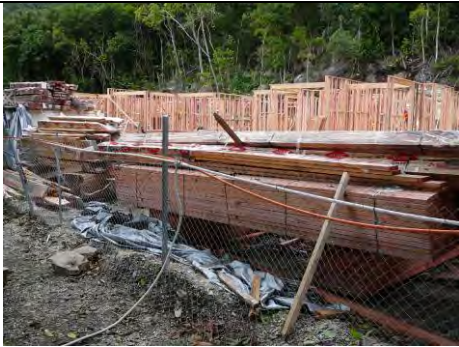
Current construction site
