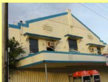
Rex Theatre façade detailing
