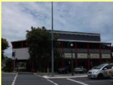
Commercial Hotel end elevation Spence St
