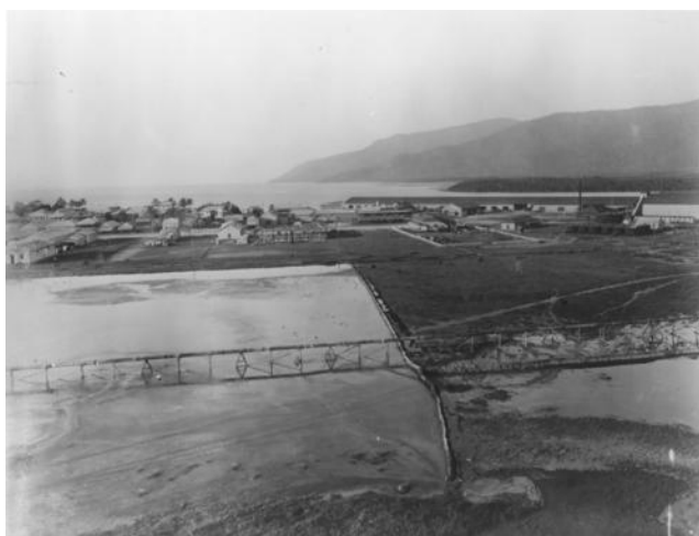
Figure 29 Mudflats below the town c1920. Crossing the picture is a pipeline on trestles and this is likely to be the sludge delivery pipe allowing areas in this section of town to be filled with the dredge from the "SD Trinity Bay". Source SLQ
