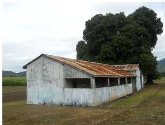
Figure 25 "Straguszi" brick cane barracks at Gordonvale. These barracks predate the introduction of associated ablutions after 1915. A shower room was subsequently installed under the right-hand side of the verandah. The building contains a kitchen but rear barrack rooms have been demolished. Source: heritage Alliance, 2011.
