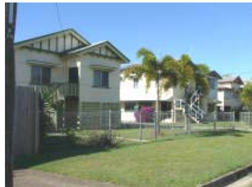
Figure 44 House at 25 Minnie Street (LHS), a Redicut form of House available as a ready to build structure railed to Cairns. Source heritage ALLIANCE 2008
