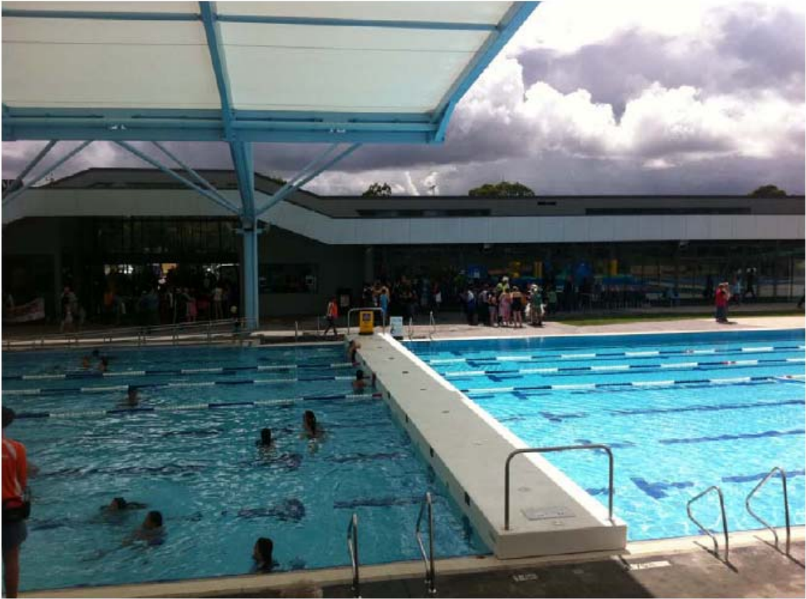
Photo 6 - Movable bulkhead in the 50m lap pool at the Nobel Park Aquatic centre in Dandenong, Victoria
