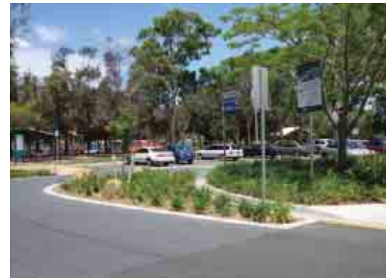
Kerbless planting beds with simple concrete edge restraints, incorporating WSUD treatments
