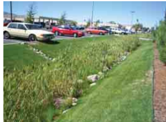
Example of swale in carpark
