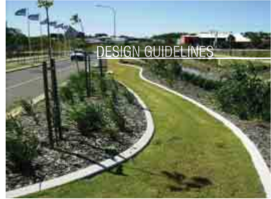
Formalised roadside WSUD
