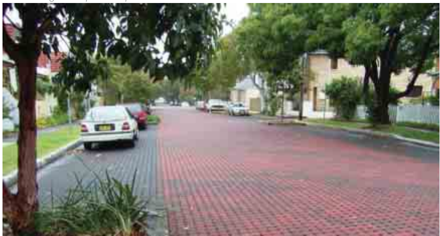
Interlocking block pavers - permeable road treatments for local streets or service access areas
