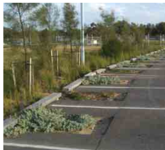
Example of WSUD incorporated with parking
