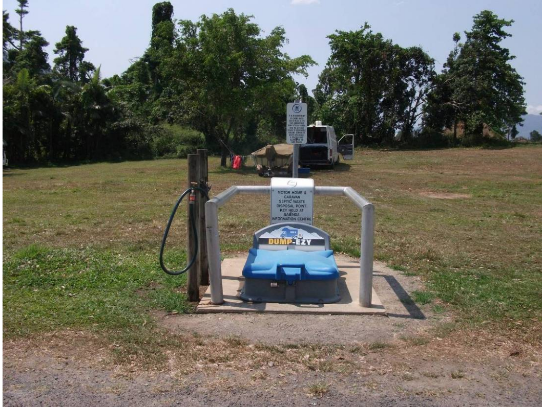
Figure 1 – Existing dump point facility
