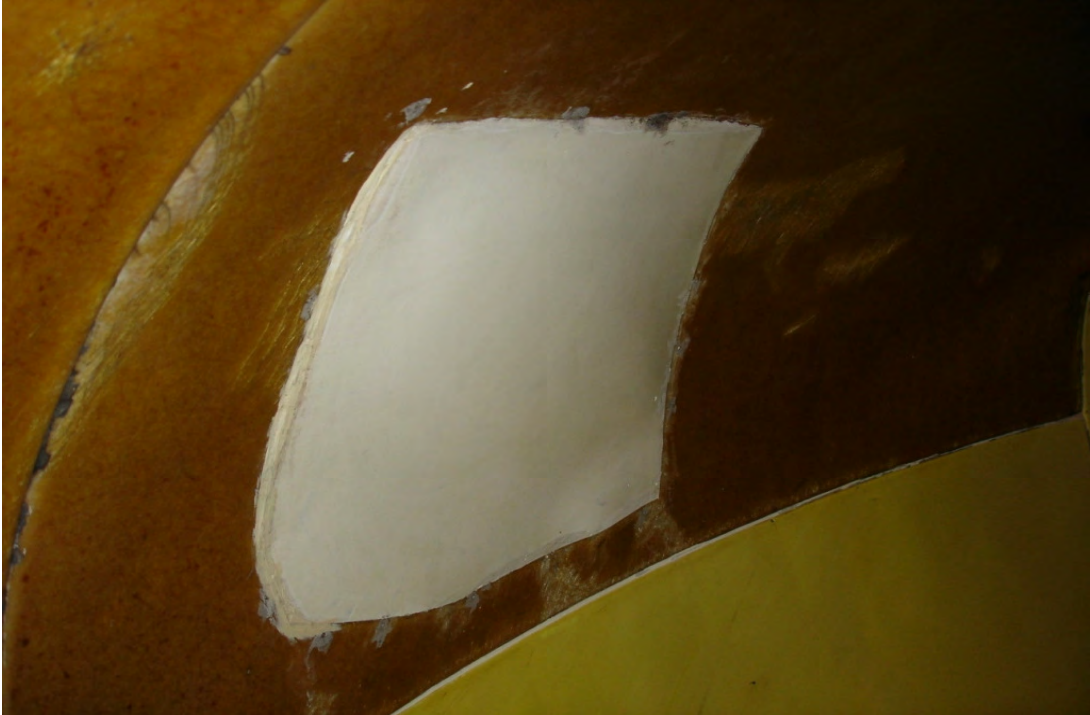
15. Patching to tubing walls
