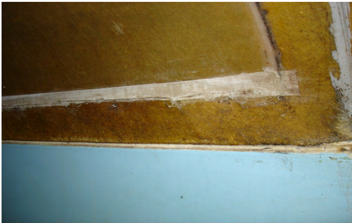
14. Patching to tubing walls
