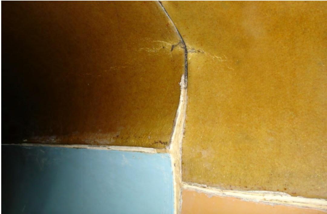
16. Inward bowing of the tubing due to overgrown tree
